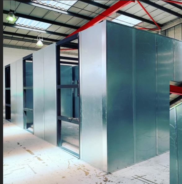
View on the rear elevation during pre build process in our factory
