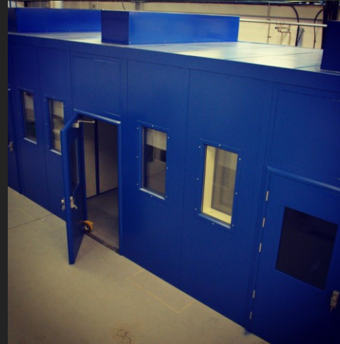
View from above showing the attenuated air intakes situated on the roof.
